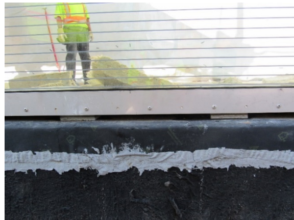
Fig. 12 Galvanized steel shims at glass shoe detail
