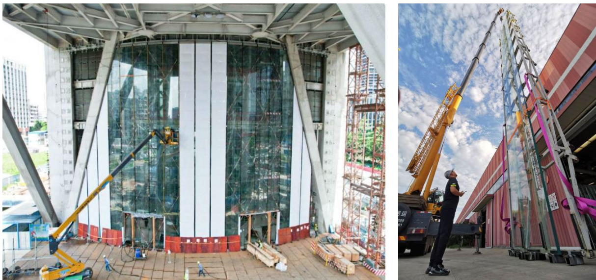
Fig. 25 & 26: Guangdong Business Center, China.
