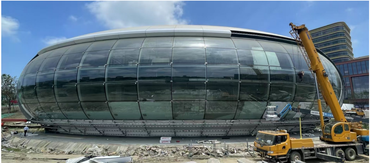
Fig. 9: Huawei “Red Bean”, China (job site).
