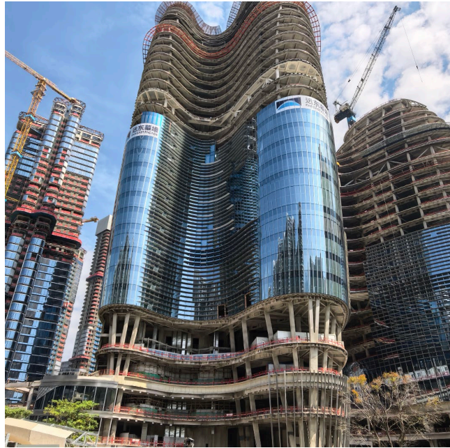
Fig. 18: OPPO Headquarters, China (job site).
