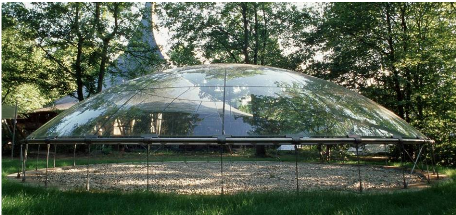
Figure 3: Prototype of a frameless glass shell built at ILEK, University of Stuttgart.
