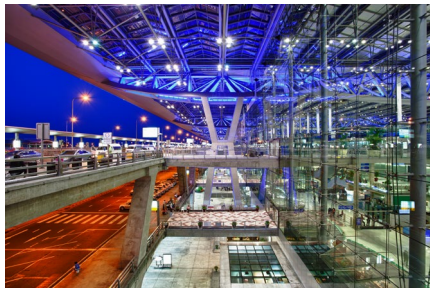
Fig. 5e: Finished project.
