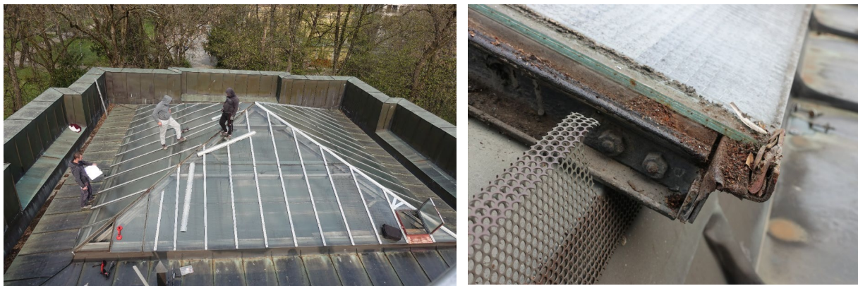
Fig. 5: Historic glass roof with wired glass.
