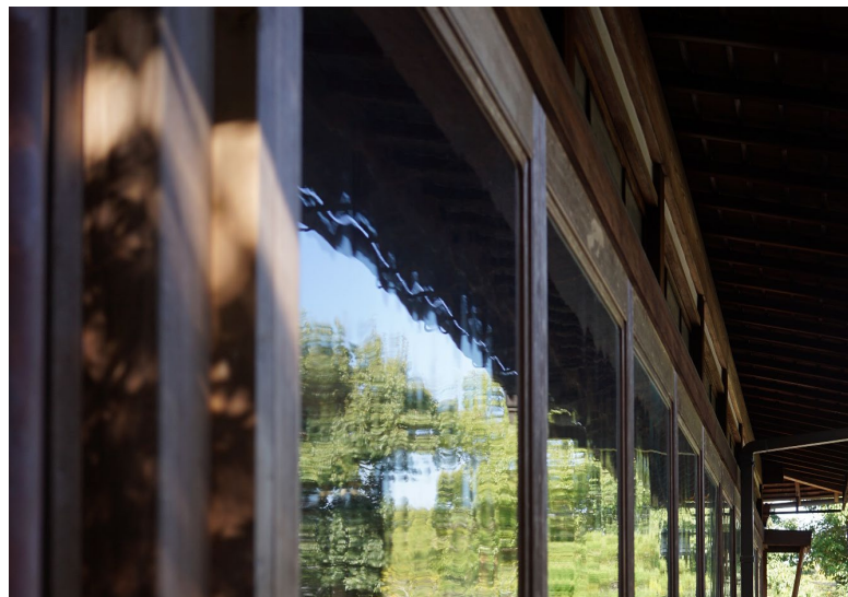
Fig. 3: Typical surface of drawn sheet glass.
