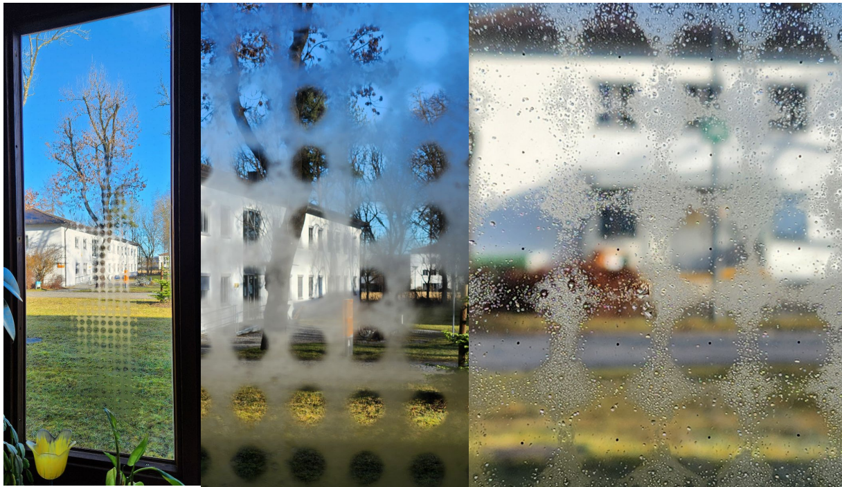
Fig. 7: Polka dots: Fogging enforced by morning dew on the outer surface of the VIG, pillars acting as thermal bridge create clear circles because local temperature is too high for dew effect. In right macro picture pillars are visible as black spots.
