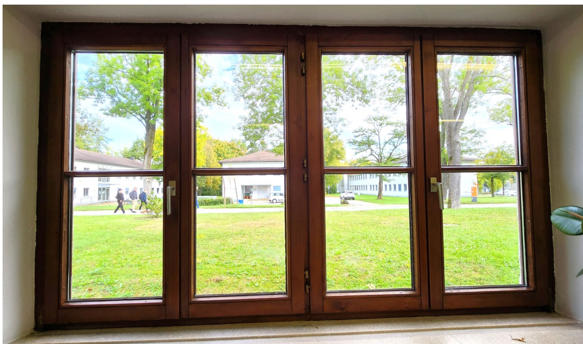
Fig. 2: Two side-by-side windows with one tilt-and-turn (outer) and one casement each with IGU before change to VIG.
