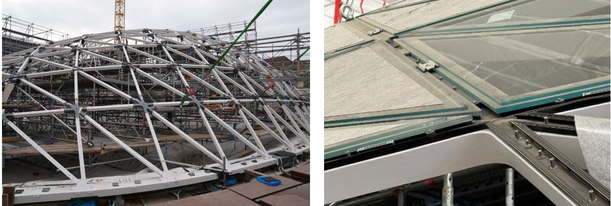
Fig. 11: Steel & Glazing work on site ©Werner Sobek AG.
