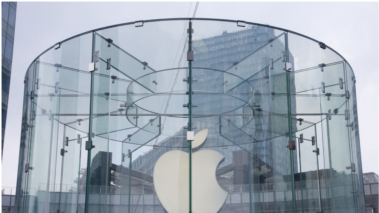
Fig. 2: Pudong Drum - Glass Frame and Mechanical Fixings visible ©EOC.
