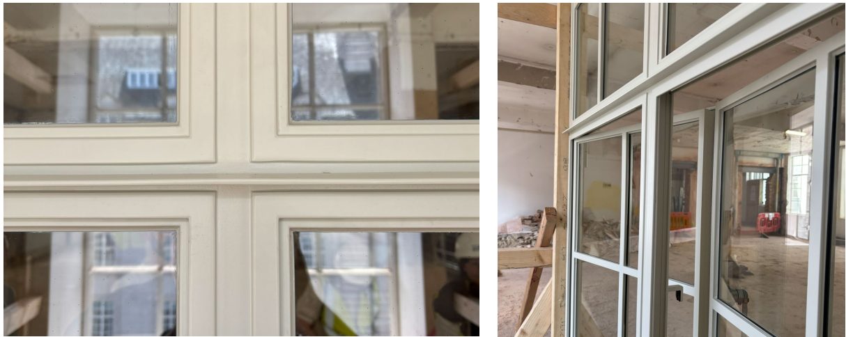
Fig. 17: Typical Regent Street window from the front (Top left) MHB-prototype window in-situ on Regent Street, bottom left window (top right), Details and demonstration of the 'hidden vent' system which allows matching the detailing and sightlines of opening vents and fixed lites, maintaining the heritage shadow lines and articulation of the framing (bottom).
