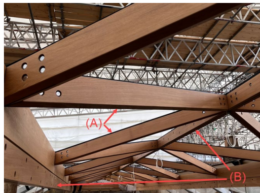
Fig. 3: Combination of the solid timber and flitch beams. (A) Solid timber beams. (B) Flitch beams. (C) Steel beams.
