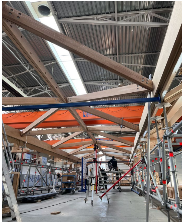
Fig. 7: Pre-assembly of the main roof at Bellapart's workshop.
