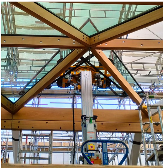
Fig. 8: Installation of the main roof.
