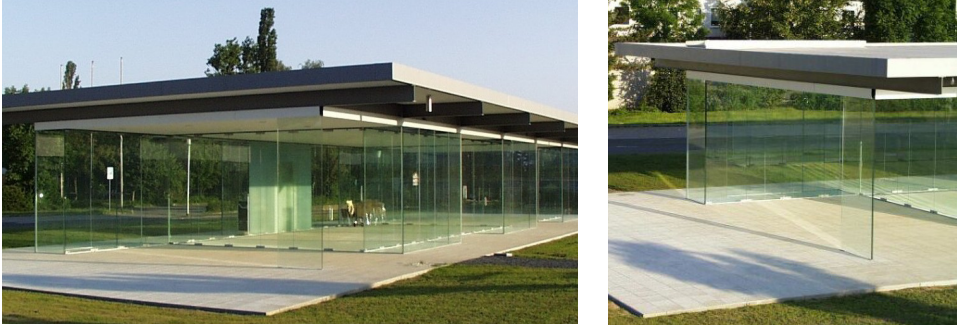
Figure 1: Application of pane-like glass columns: Glaspavillon Rheinbach (D).
