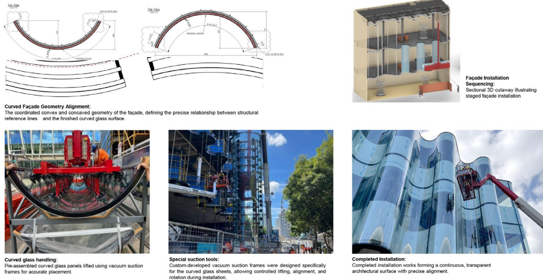
Fig. 3: Glazing Installation.
