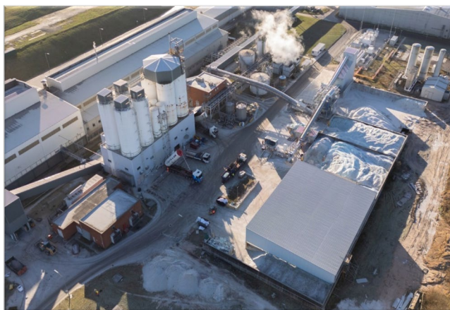
Fig. 7: New Cullet Reprocessing Facility (2023).
