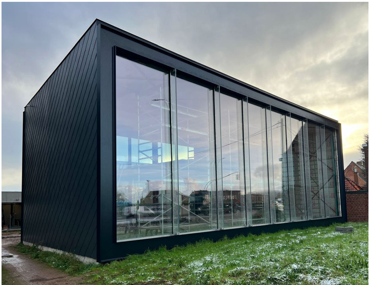
Fig. 3: Front and rear façade.
