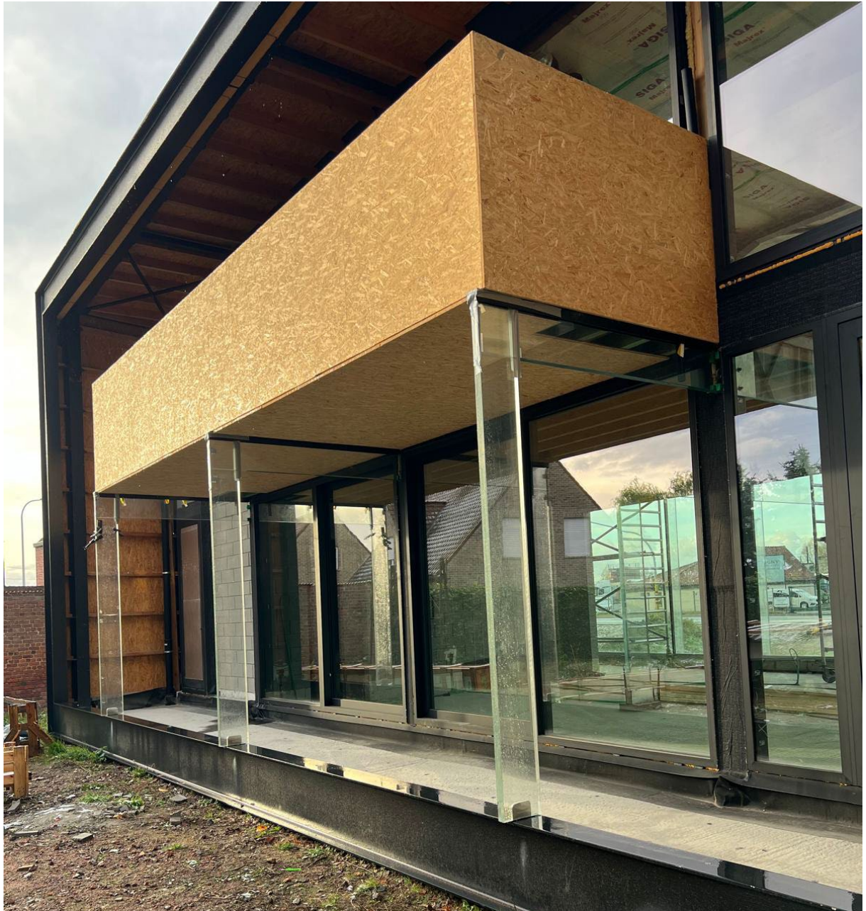
Fig. 2: Structural glass features in the Glass Quarters .
