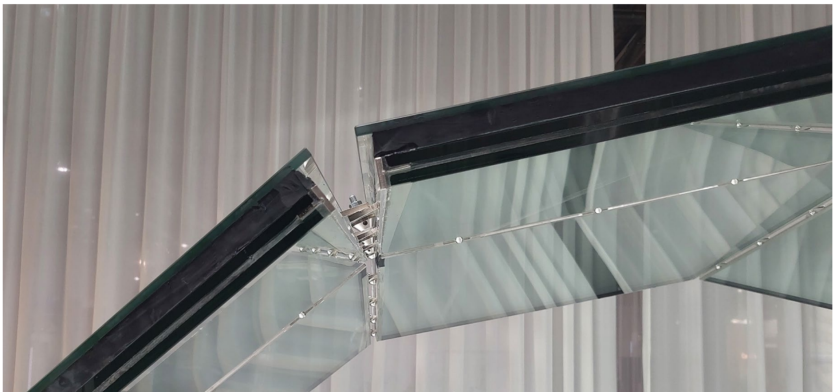
Fig. 18: Close-up of the construction detail and fittings produced for the Glasstec mock-up exhibited in Düsseldorf in 2024 (Source: knippershelbig).
