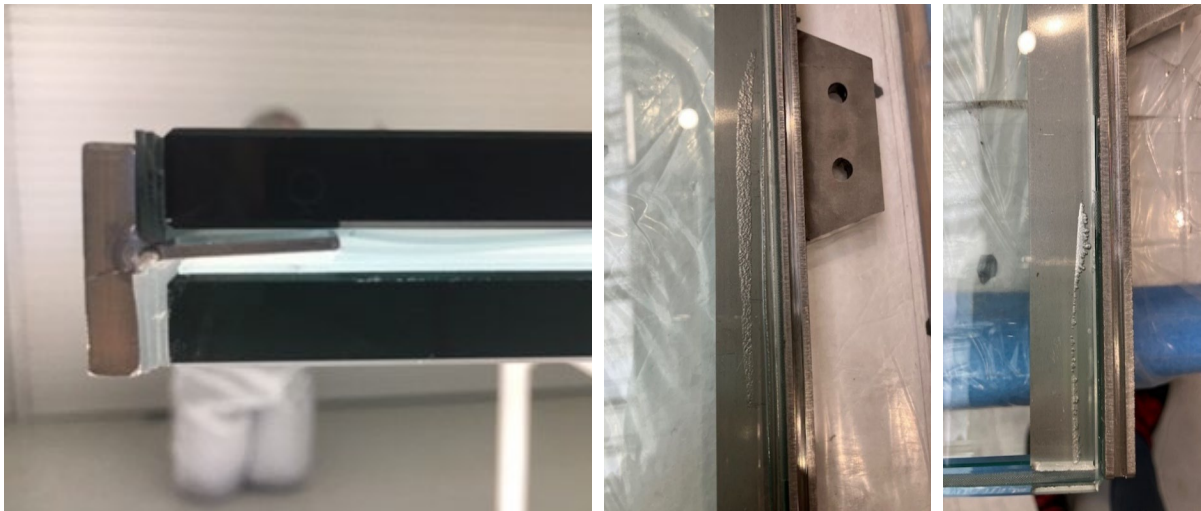
Fig. 3: Example of laminated non-orthogonal steel fitting (left) and resulting air entrapment (middle and right) (Source: Yachtglass).
