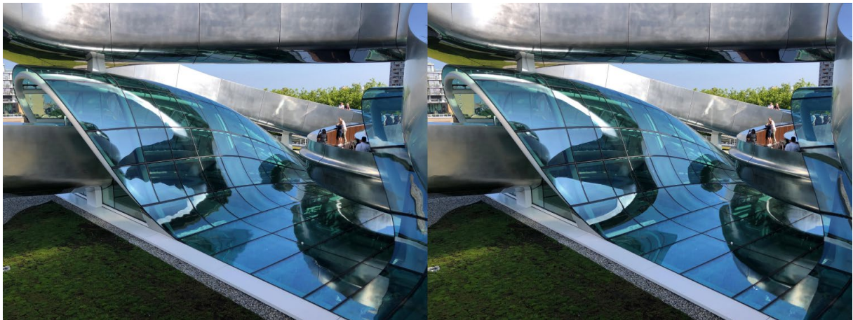
Fig. 11: Potential difference in optical surface quality between hot bending (left) and cold bending (right) (own work, 2025)
