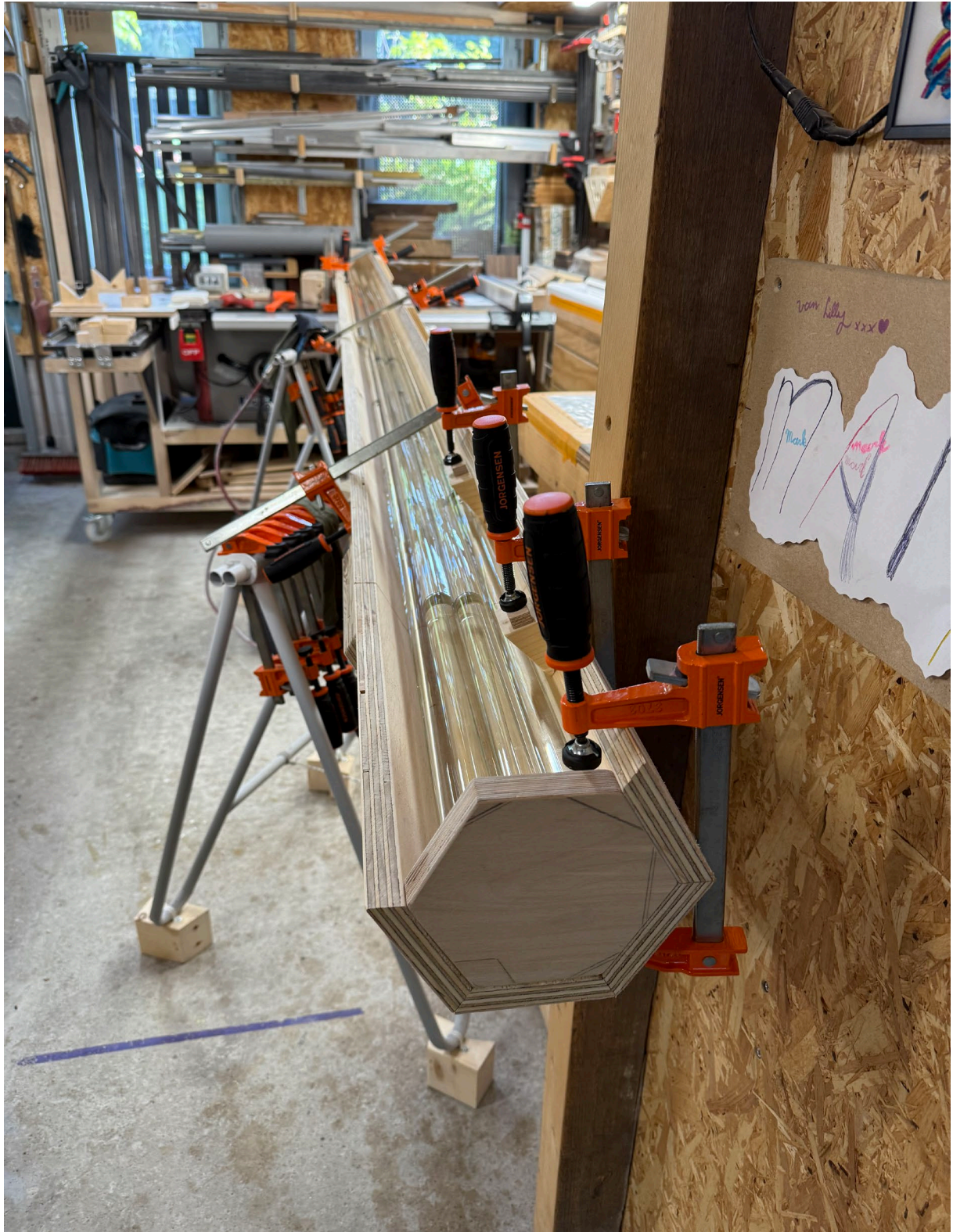
Fig. 7. Production of the hexagonal glass column in the workshop of G&SS in Rotterdam.
