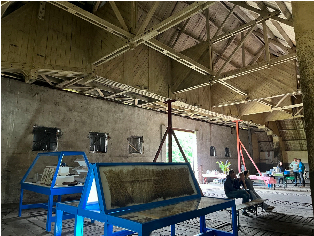
Fig. 2. The two temporarily steel support structures (in red) in the hangar during an exhibition about bio-based building materials.
