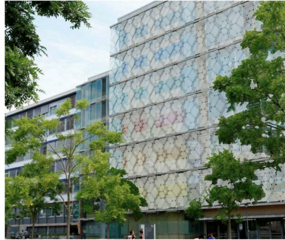
Fig. 5: Folded glass façade structure connected using zippers © Bouwman, Klein, Kujus.
