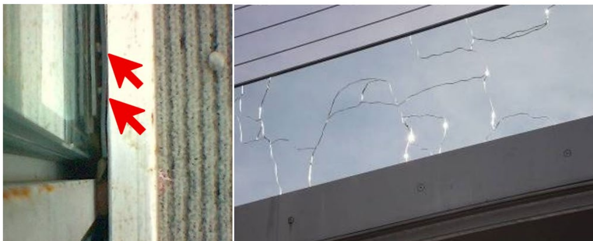
Fig. 5: Sand, gravel and particles in the clamping insert area.
