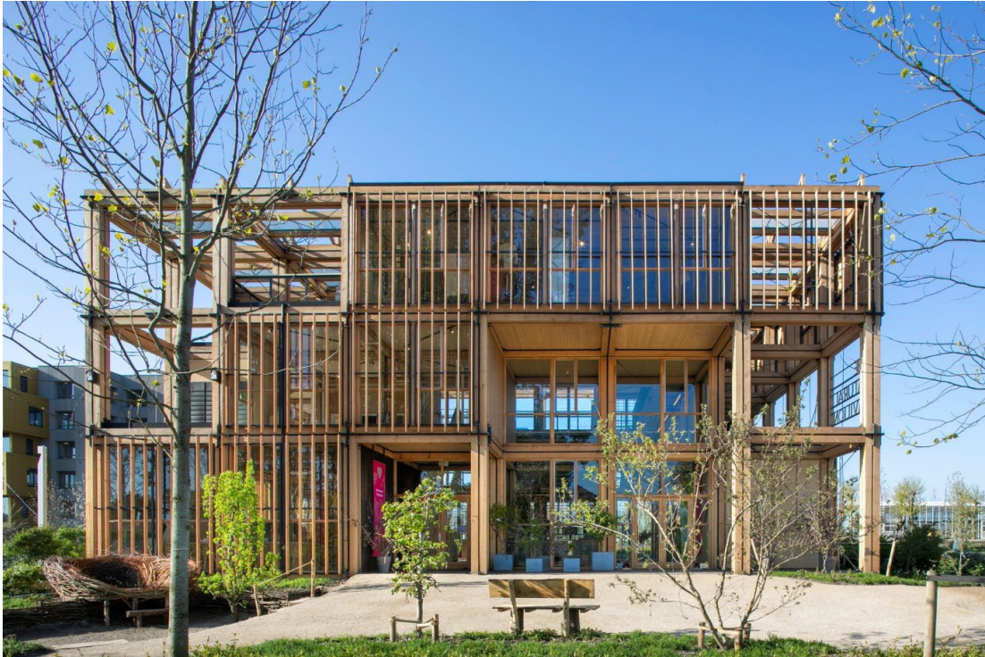
Fig.1. The Natural Pavilion (photographed by Scagliola, D., Brakkee, S.).
