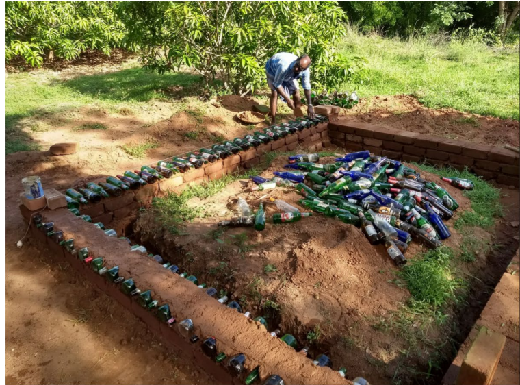
(b) Construction method
