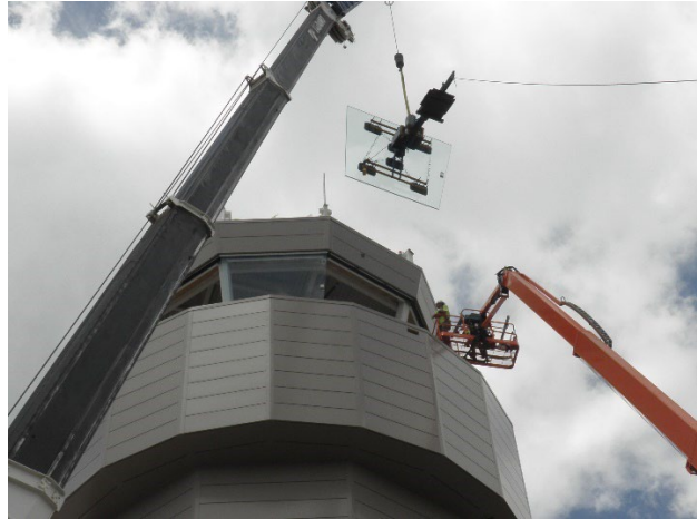
Fig. 5: Sarasota Installation – Key Glass.
