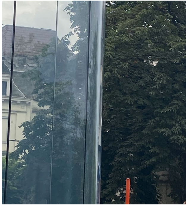
Fig. 1: Effects of haze on the background. In the image, the effect is amplified as the background is seen through two layers of hazy glass.
