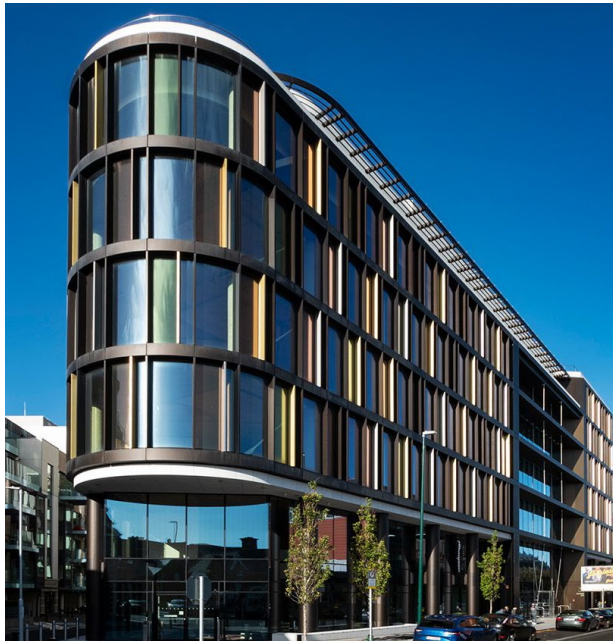
Fig. 2: IPC House, Dublin – curved SSG (GLF Facades).
