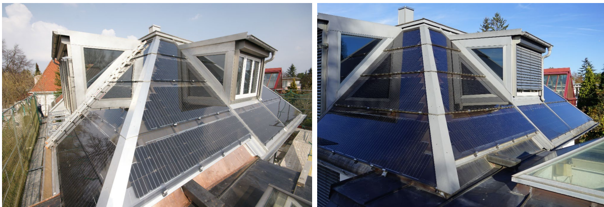
Fig. 11: Fig. 3: Photovoltaic roof in Munich 2012 (left) and 2022 (right).
