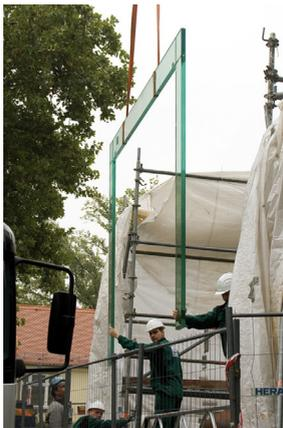
Figure 8: Glass frame erection.
