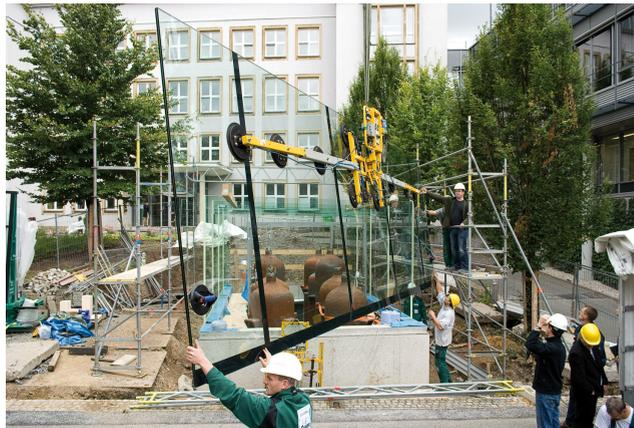
Figure 9: Installation of the large-sized lateral glazing.
