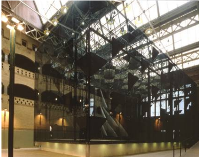
Figure 1: Outside view of the Glass Music Hall of 1990 designed by Cees Spanjers and Mick Eekhout.
