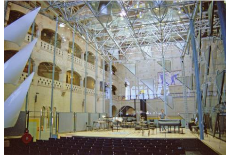
Figure 2: Inside view of the Glass Music Hall of 1990 designed by Cees Spanjers and Mick Eekhout.
