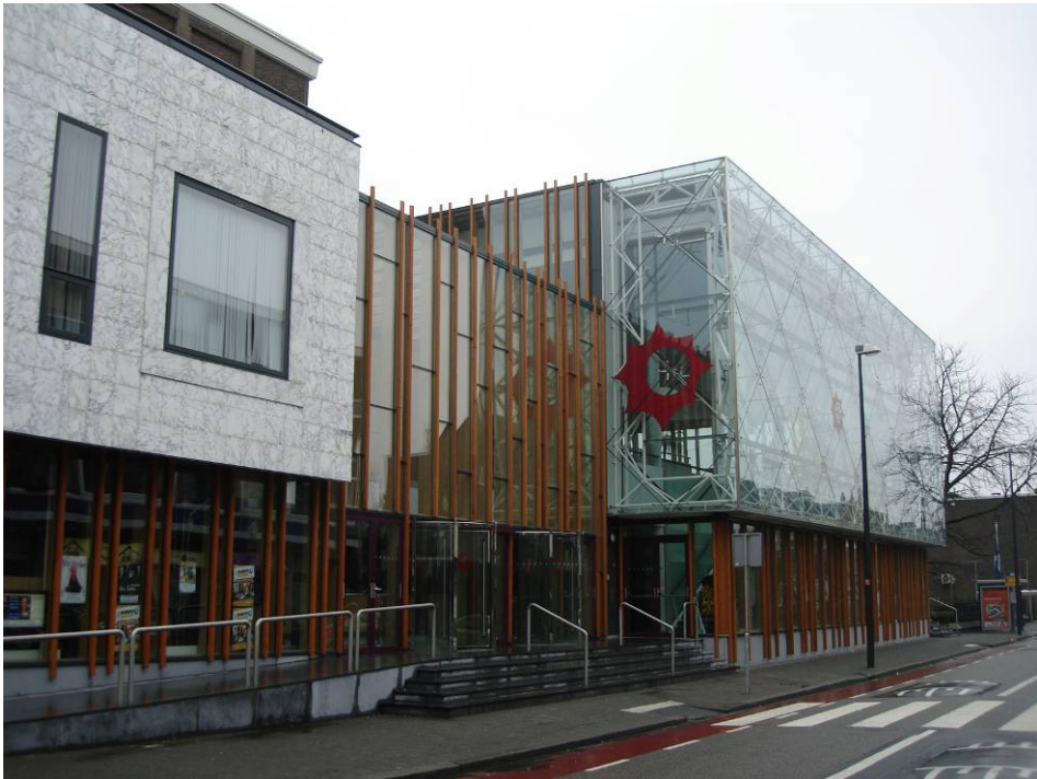
Figure 18: View of the structure.
