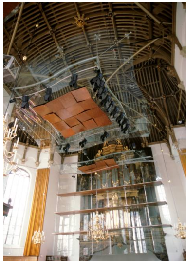
Figure 3: interior view of the suspended glass envelope in the Nieuwe Kerk, The Hague.
