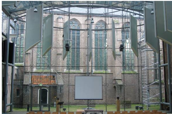
Figure 9: Prinsenhof Hall, Delft, diagonal bracing.
