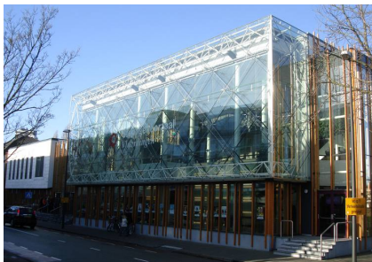
Figure 16: Exterior view of the façade.
