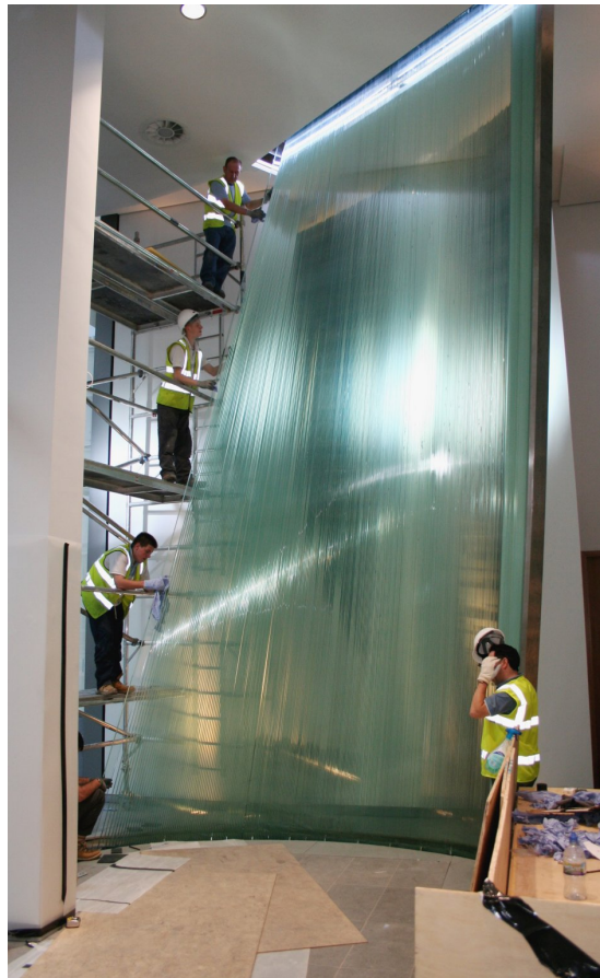
Figure 14: Installation of 'Veil', London.
