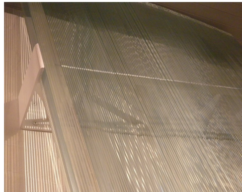
Figure 11: End support to glass beam.
