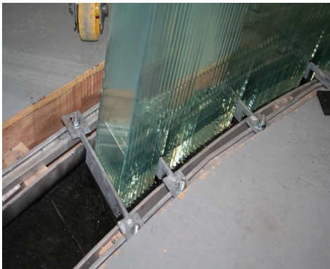
Figure 10: Rotational restraint provided in base detail.
