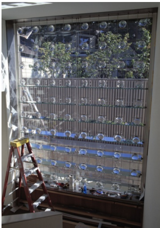
Figure 8: view of the window during installation.
