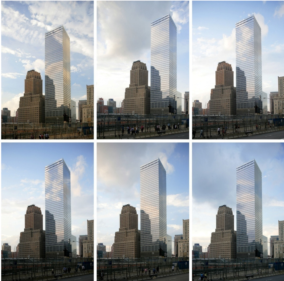
Figure 13: the 7 World Trade Center curtain wall responding to the sky conditions.
