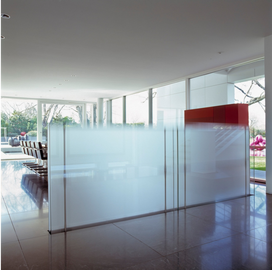
Figure 2: view from the gallery of the “Retracting Screen” as it descends into the floor.
