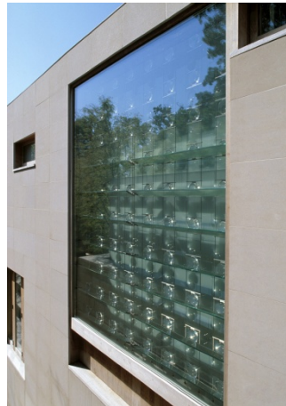
Figure 9: the completed window seen from outside.
