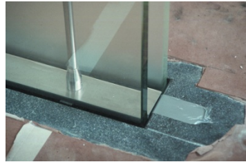
Figure 5a, b, c: details showing the center rods, glass connections, laminated panels and base beam.
