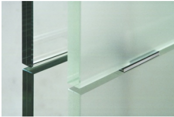
Figure 5a, b, c: details showing the center rods, glass connections, laminated panels and base beam.
