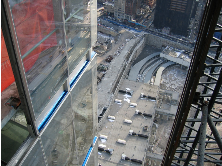
Figure 15: view of the blue reflectors during installation.
