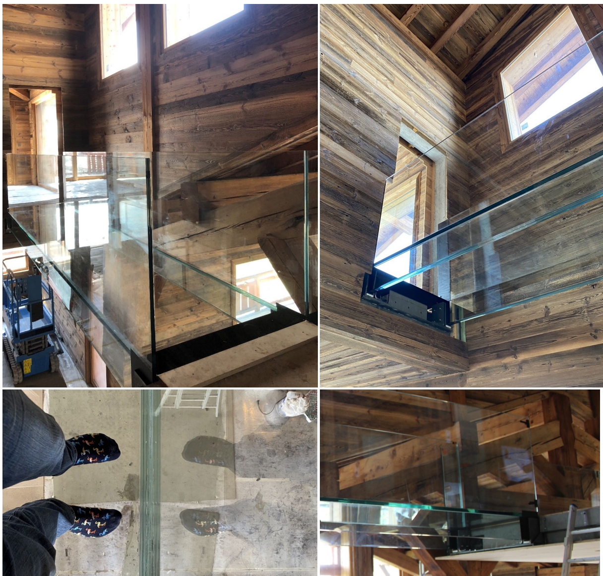
Fig. 6:all-glass walkway after completion.
