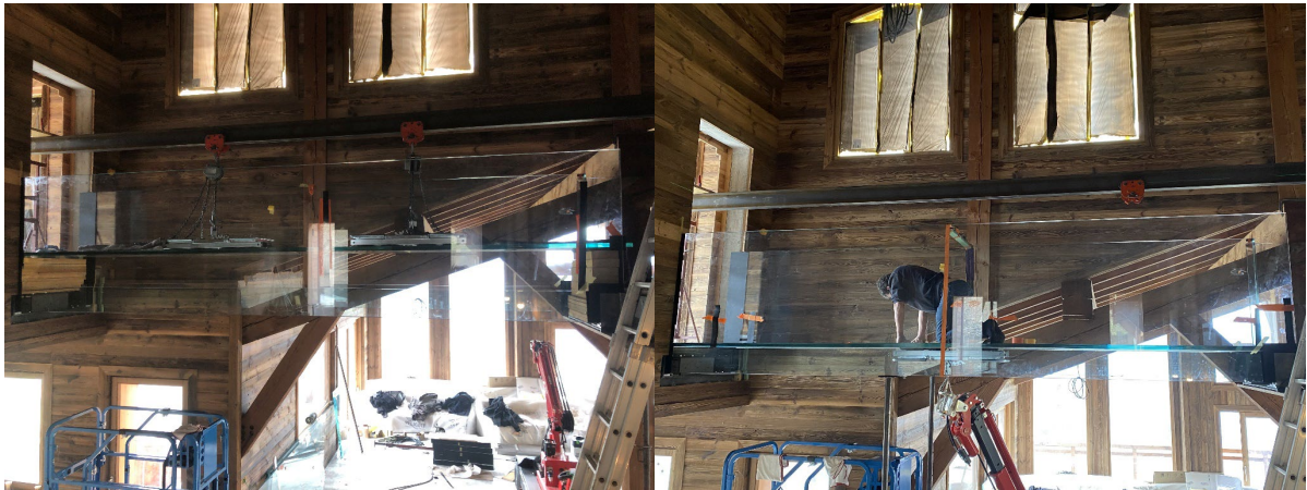
Fig. 5:all-glass walkway during construction.
