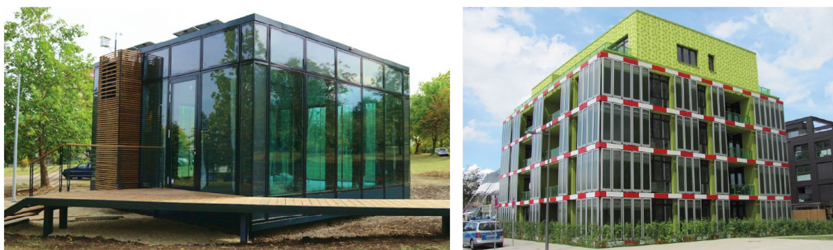
Fig. 1: Pilot projects. Left) Demonstration pavilion with a thermally regulated fluid in the pane cavity (InDeWaG 2023) Right) BIQ with photobioreactor façade (Energie Zukunft 2020).
