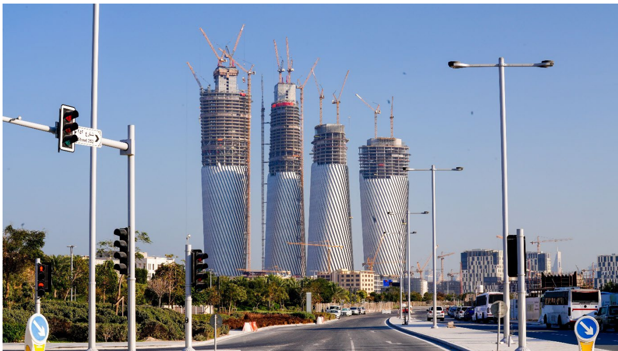
Fig. 1: Aerial view of the project, under construction.
