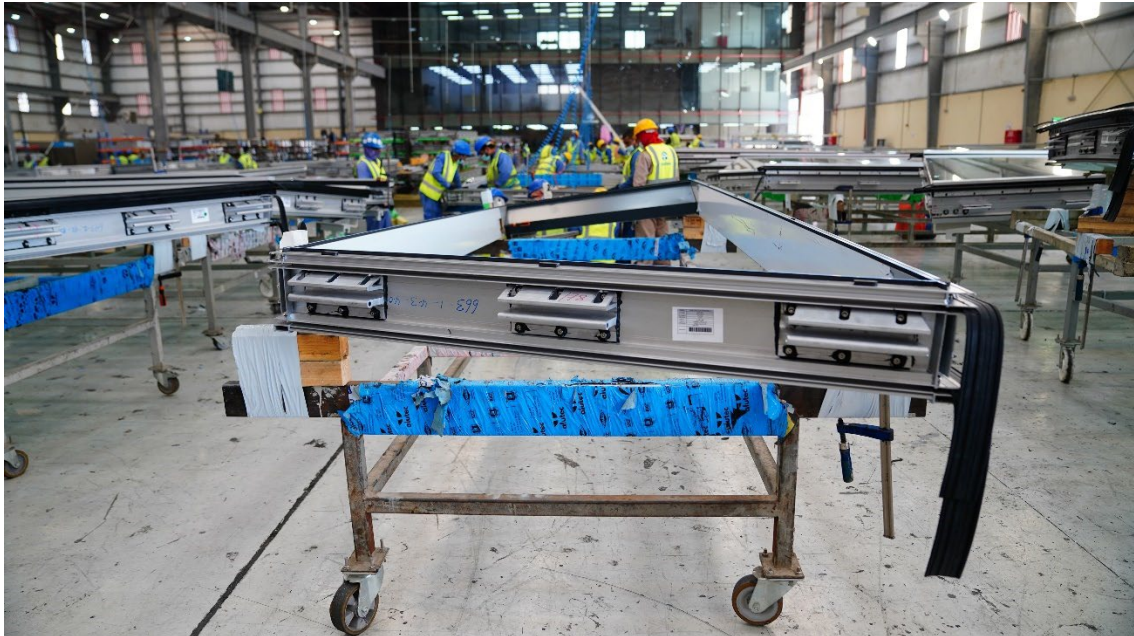
Fig. 7: Curtainwall unit pre-assembled in its final 3D geometry.
