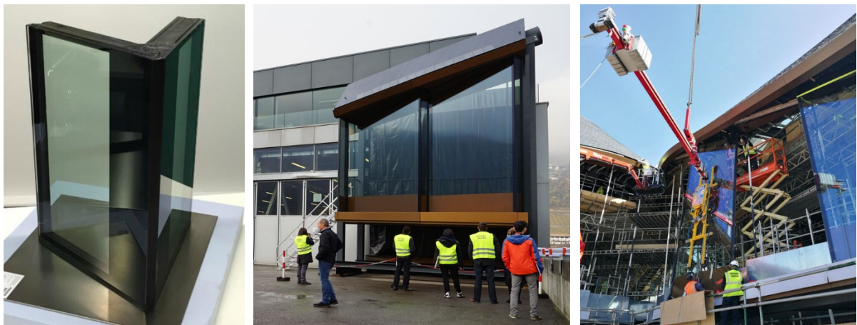
Fig. 11: Left- Hand mock up of connection, Middle – Visual mock up, Right – Project during façade installation
