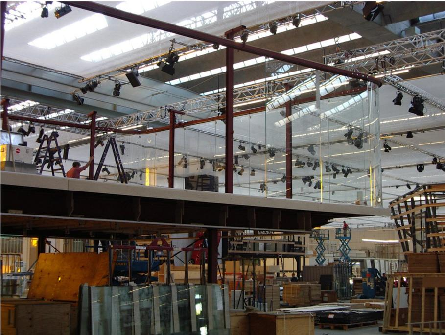
Figure 8: Steel frame with mike booms and mounted glasses at the narrow side.
