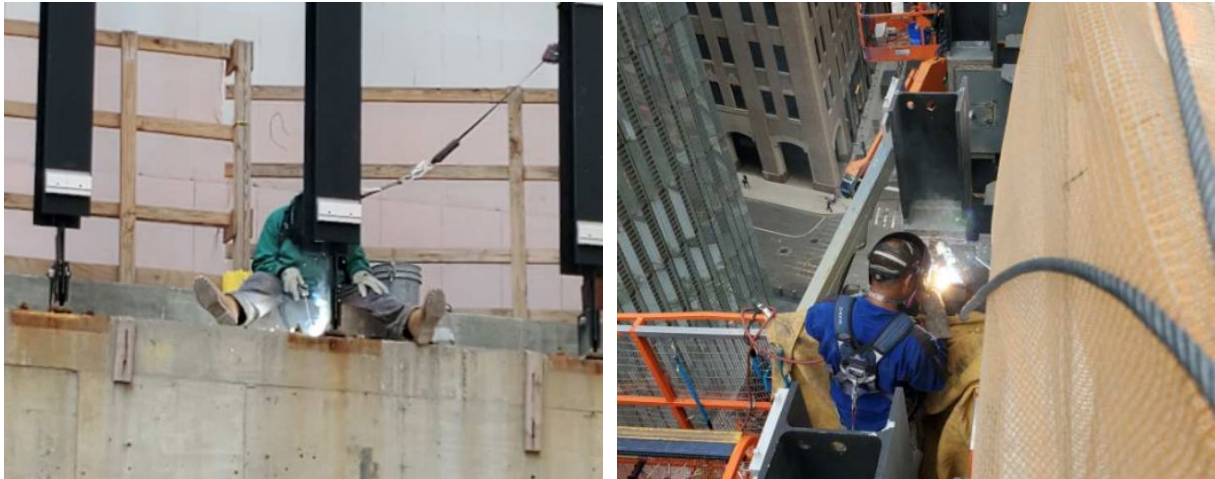
Fig. 8: On-site welding. ©Josef Gartner GmbH
