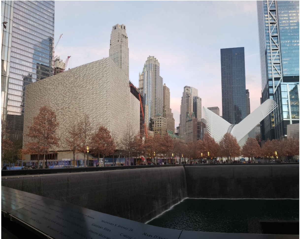
Fig. 11: Final Steps of Installation at the North Wall seen from the WTC Memorial. ©Josef Gartner GmbH
