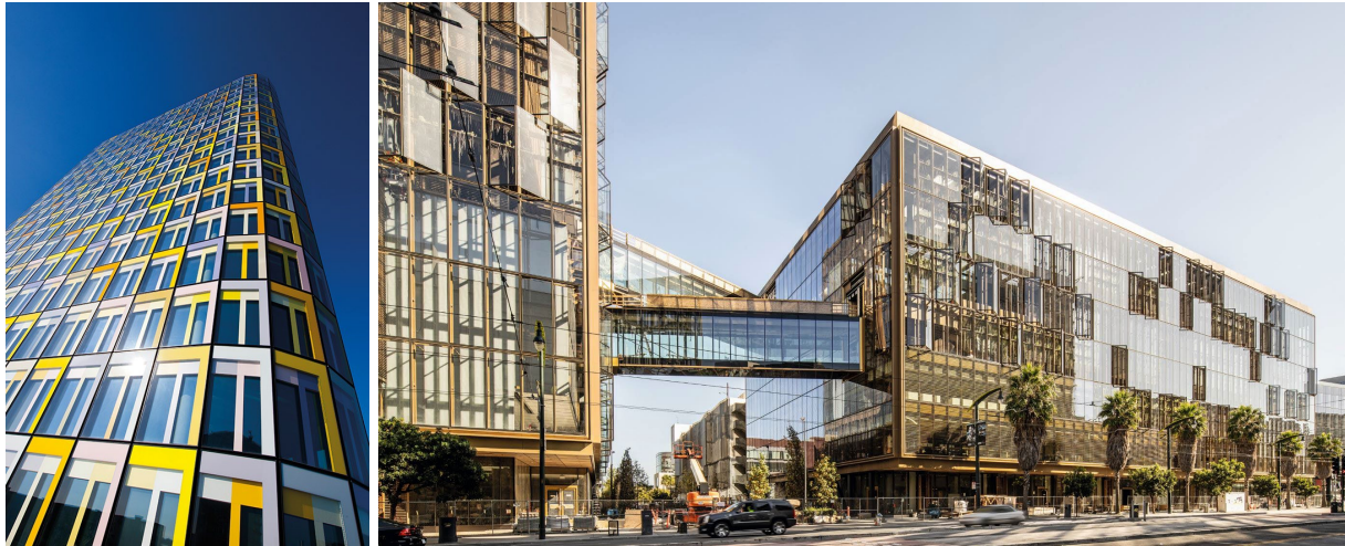
Fig. 5: Double-Skin Facades at ADAC, Munich (left, ©Stephan Liebl) and UBER, San Francisco (right, ©Jason O'Rear Photography).
