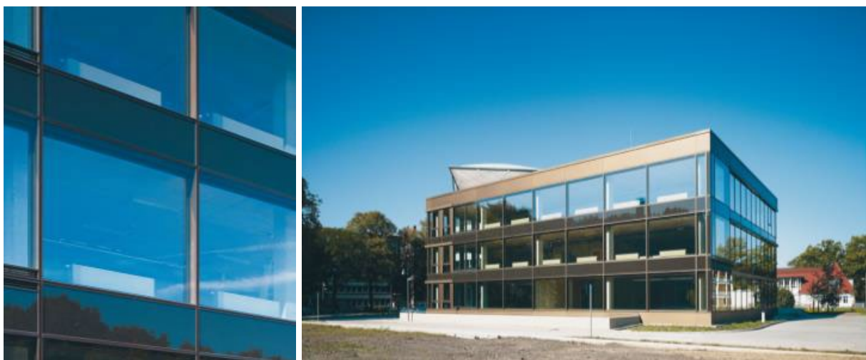
Fig. 3: First Closed-Cavity Facade at InHaus 2, Duisburg. ©Guido Erbring Architekturfotografie
