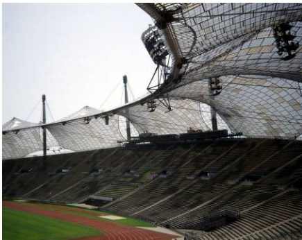
Figure 2: Glass roofs Olympic Stadium by Günther Benisch and Frei Otto
