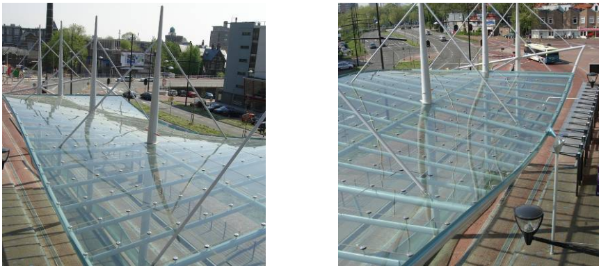
Figure 14: Glass roof from above
