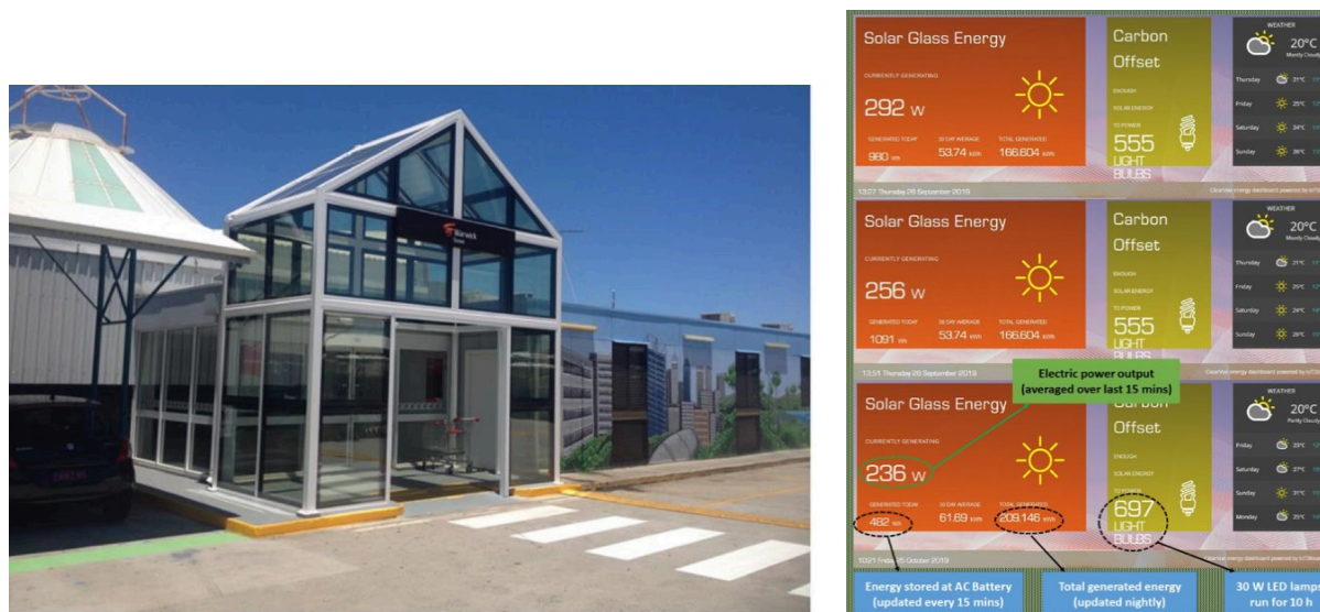
Fig. 2: Warwick Grove Shopping Centre Atrium (Perth, Australia) built using Clearvue solar windows and a summary of measured solar installation performance (18 multi-oriented solar windows in total).
