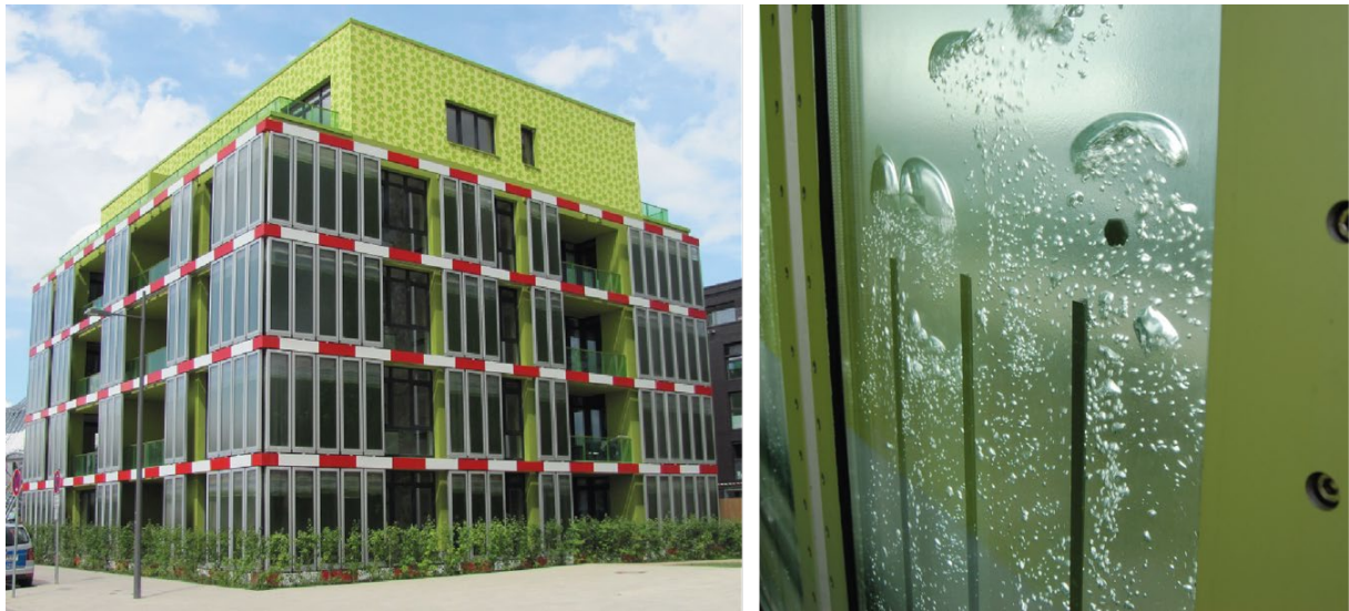
Fig. 2: BIQ algae house with photobioreactor façade.
