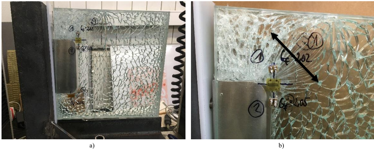
Fig. 8 a) Crack pattern on inner glass ply and b) detail of crack pattern above embedded insert.
