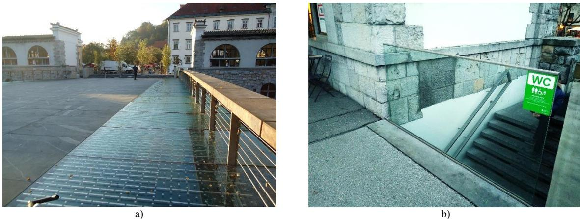
Fig. 1 Butchers' bridge with laminated glass bridge deck over the river Ljubljanica in Ljubljana a) and laminated glass balustrade b).
