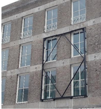
Fig. 13 frame to check dimensions existing façade.
