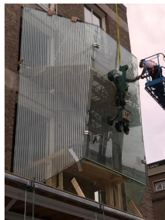
Fig. 18 installation of front panel.
