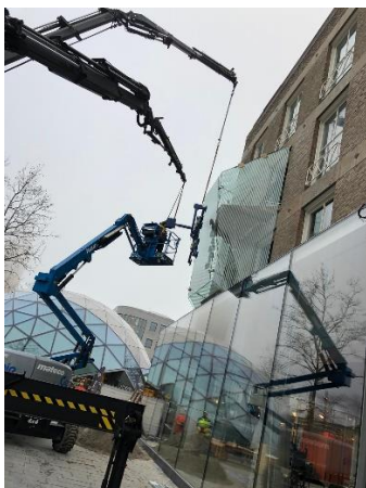
Fig. 17 installation of front panel.
