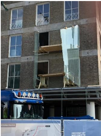
Fig. 15 installation of side panels.
