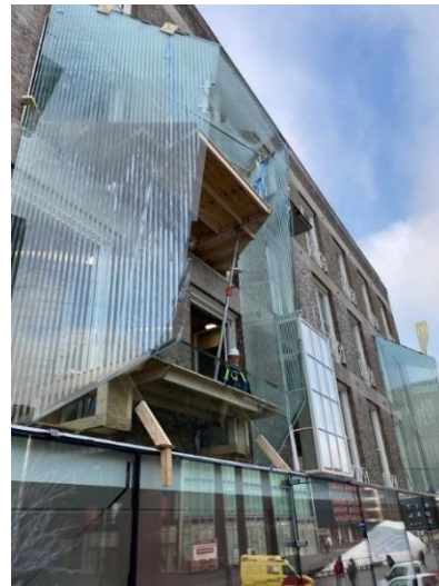
Fig. 16 installation of top panel.
