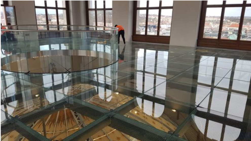
Fig. 12 Finally cleaned structure ready for service.
