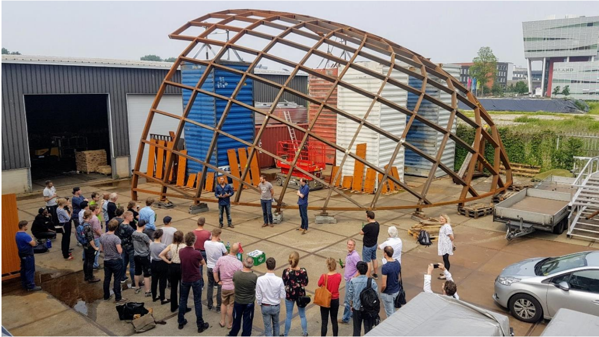
Fig. 13 Test-assembly steel pre-assembled frames.
