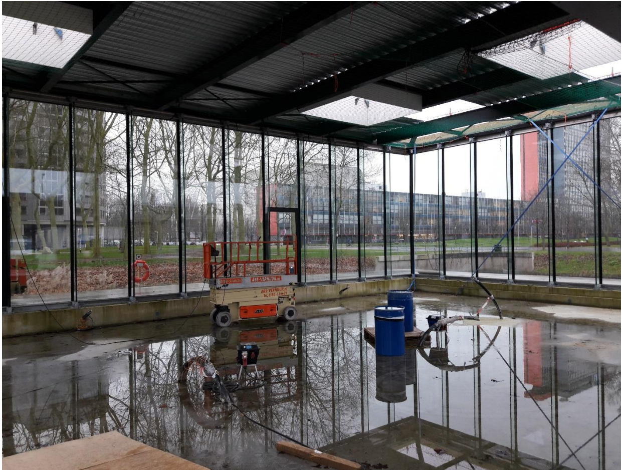
Fig. 12 Co Creation Centre during installation in January 2020.
