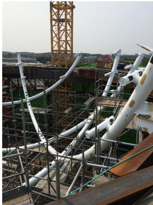
Fig. 2 Main ring supports.
