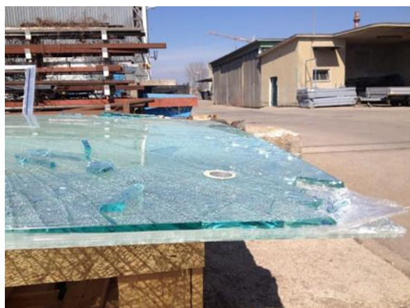
Fig. 5 Delamination after breakage.
