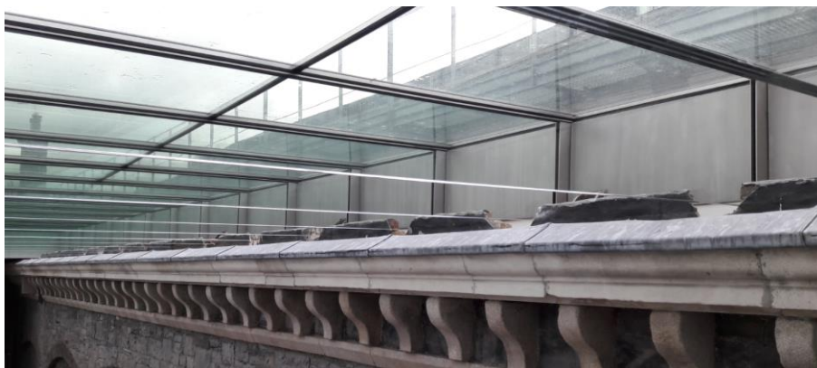
Fig. 24 Glass on installed on site.
