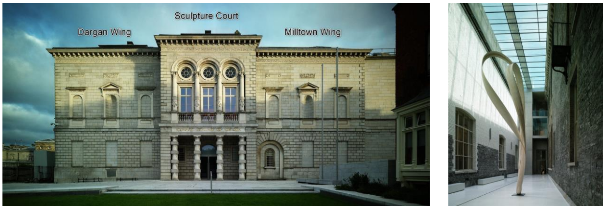
Fig. 13 (Left) National Gallery of Ireland, seen from the Merrion Square. (Right) Inside the courtyard (source: Marie Louise Halpenny).
