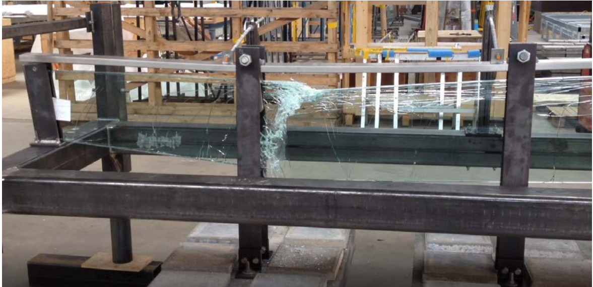
Fig. 11 Cracks in the glass fin during post breakage load test [Octatube].
