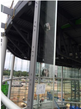
Fig. 15 Construction photo of fin splice.
