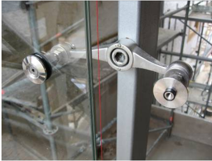
Figure 4: point fixing with tolerance compensating „spider“ which is fixed to superstructure. Figure 5: point fixed canopy with solar panel
